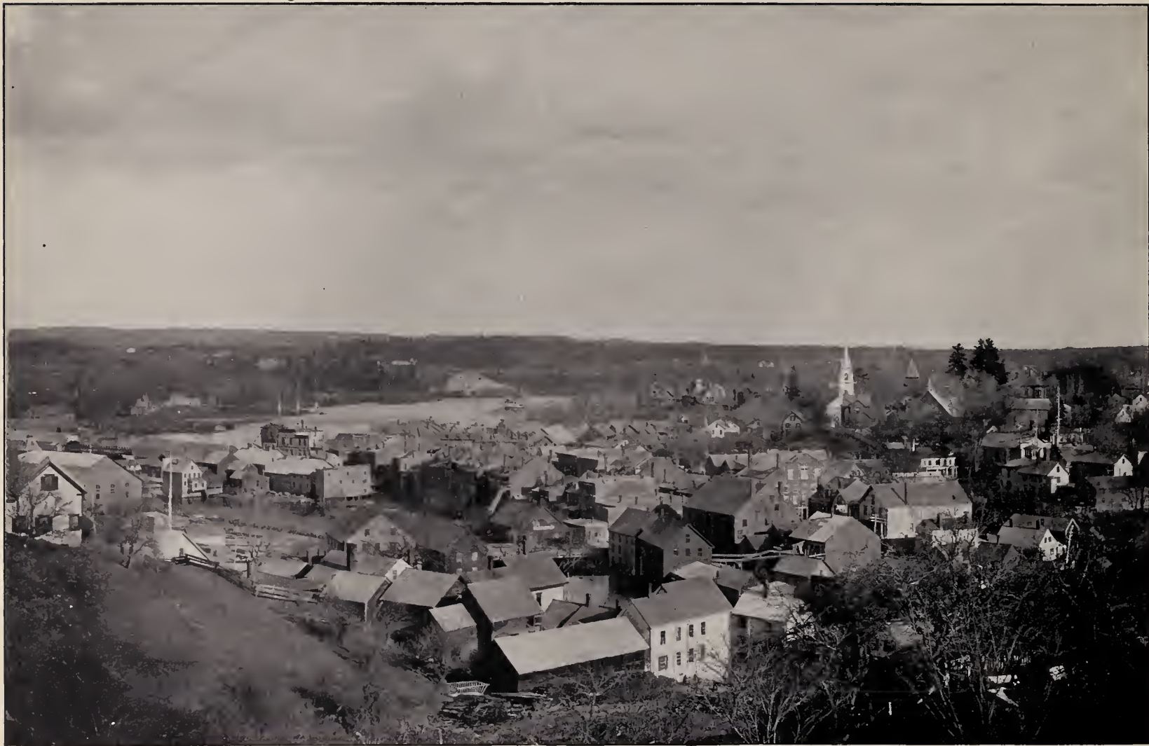
OVERLOOKING DAM NO. 1 AND LOWER WATER STREET FROM HIGHLAND AVENUE.
